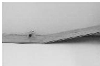
With the panel properly prepared, always lay planks from left to right, groove profile facing away from the wall. To join the second plank in the first row to the first plank, position the tongue end over the groove end of the first plank and insert the tongue at a slight angle. A slight downward “wiggle” motion locks the planks.
