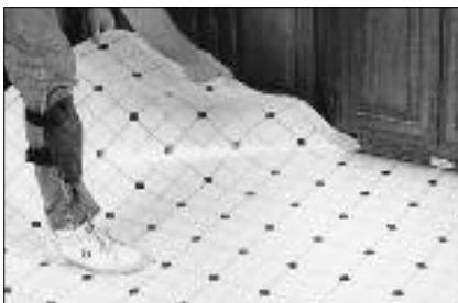
Now that the transfer and cutout are complete, the material is ready to be installed. The floor covering is an exact duplicate of the floor, with all excess material removed and all cuts made for possible obstacles. Place the material into the room and fasten as required.
