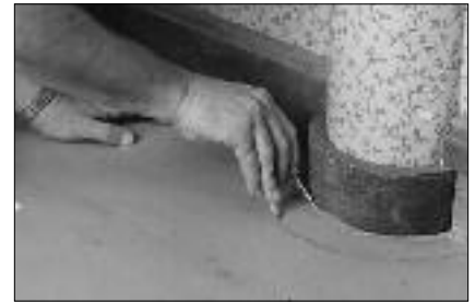
Pencil dividers make it easier to scribe irregular-shaped obstacles. Keep the dividers at a 90° angle to the item being scribed in order to keep the scribe accurate.
