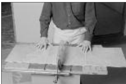
The tile panels can be cut using traditional cutting tools such as hand saws, jig saws, circular saws, power miter or chop saws, etc. The wide panel width of NatureForm Tile can be effectively cut to length using a table saw.
