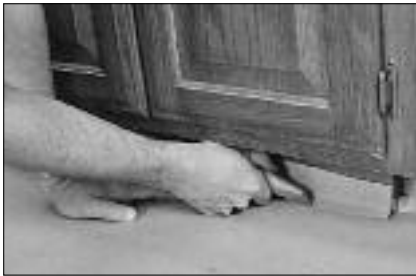
After all preparation is complete, place scribing paper on the area to be covered. Place the roll-set (curl) downward to make paper positioning easier.
