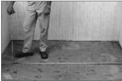
Measure out the entire work area to ensure proper panel layout. Keep in mind the last panel to be laid in the work area must be at least 3" wide. A calculator may be helpful when figuring out how to arrange the floor. A NatureForm Laminate Tile panel measures 15-3/4" wide.
