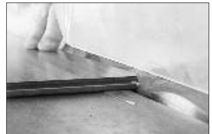
Cut off all milled profiles from the edges abutting vertical surfaces. This provides a solid edge to receive spacing devices.
