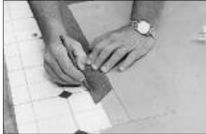
Using the same roofing square or dividers, transfer the marks on the pattern to the sheet goods, making a perfect duplicate of the floor. Be sure to keep the dividers set to the same measurement you started with and use the same leg of the square you used to make the pattern. To ensure correct pattern transfer, the person who performed the pattern scribing should also transfer the pattern onto the resilient flooring.
