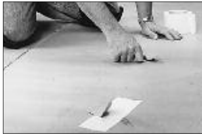
Cut windows in the paper to expose the subfloor and then use masking tape to hold the paper in place. Paper should be rough-trimmed using a utility knife to 1" from all obstructions.
